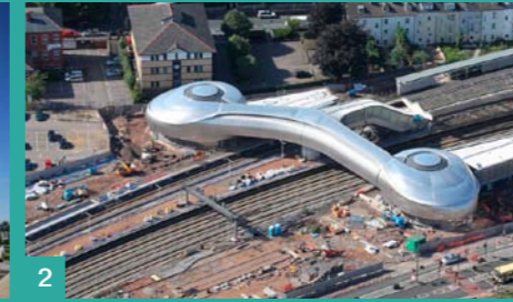
1. Wales 1 Business Park, Magor, Courtesy of Charnwood. 2. Newport Station, Courtesy of Network Rail.
