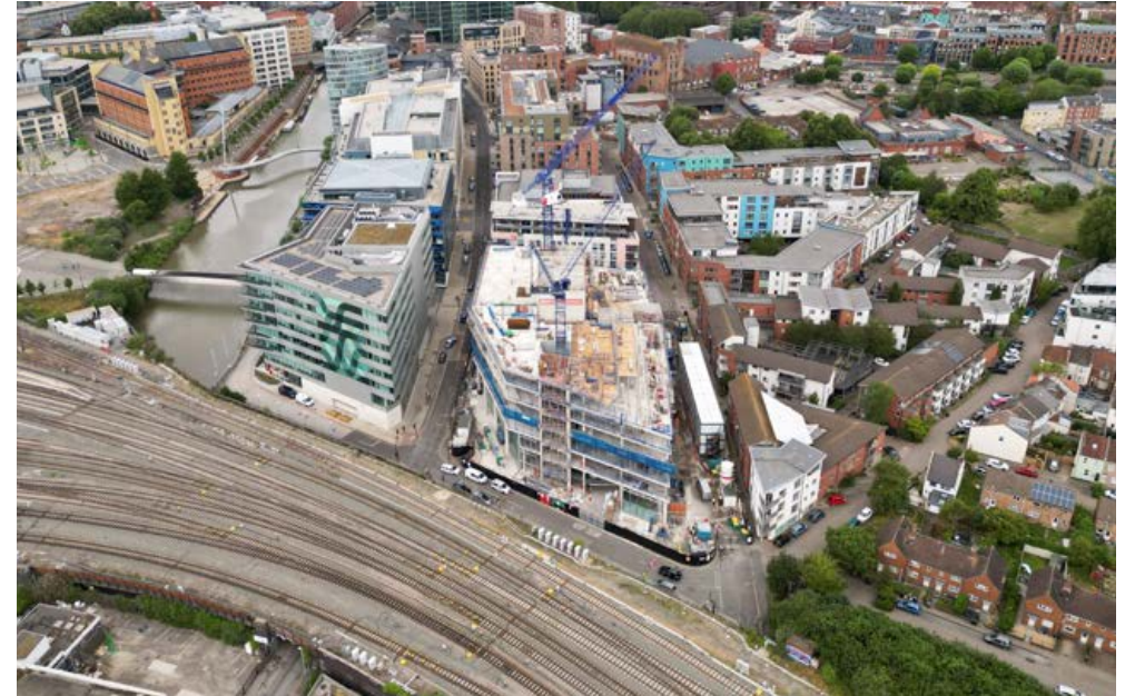
Welcome Building under construction, Avon Street, Bristol.
