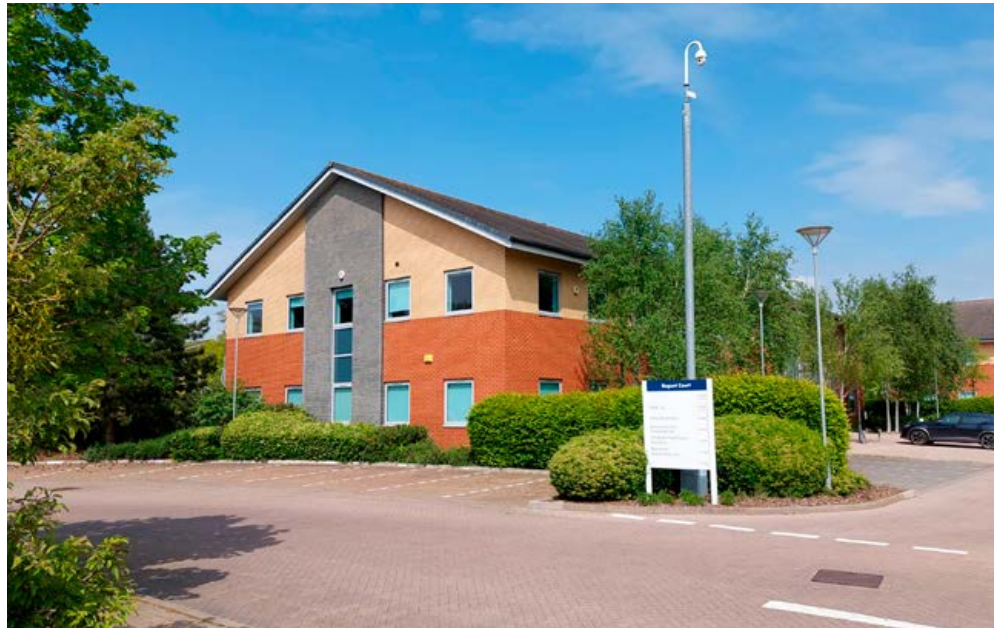
Regent Court, Gloucester Business Park.
