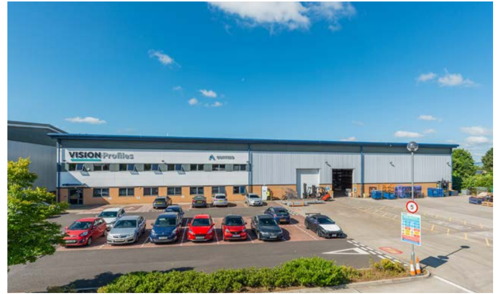
Vision Profiles, Quedgeley West, Gloucester.
